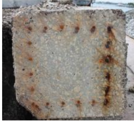
Figure 10. Submerged (i.e., bottom) end of pile from Bridge B, end view. Note that the absolute bottom end of the in-service pile was left in situ and that this pile portion was cut from it.
