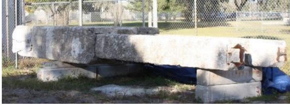
Figure 1. Bridge A piles resting side-by-side on horizontal concrete columns. Note jackets on upper area (left) of piles and H-beams visible at each pile bottom end (right).
