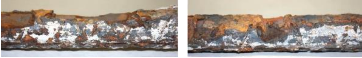
Figure 16. Severe localized corrosion-related cross-section loss, Bridge A. Corrosion was limited to relatively short segments of the bar length and in each segment most of the metal loss took place on the side of the bar facing the external pile surface (top of each picture). Bar #2a; locations from left to right: 140 and 175 in (3.6 and 4.4 m) below high tide, respectively. The rebar is 1 in (2.5 cm) in diameter.
